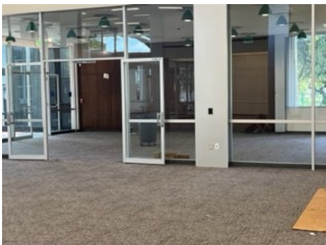
Left, future library room.
